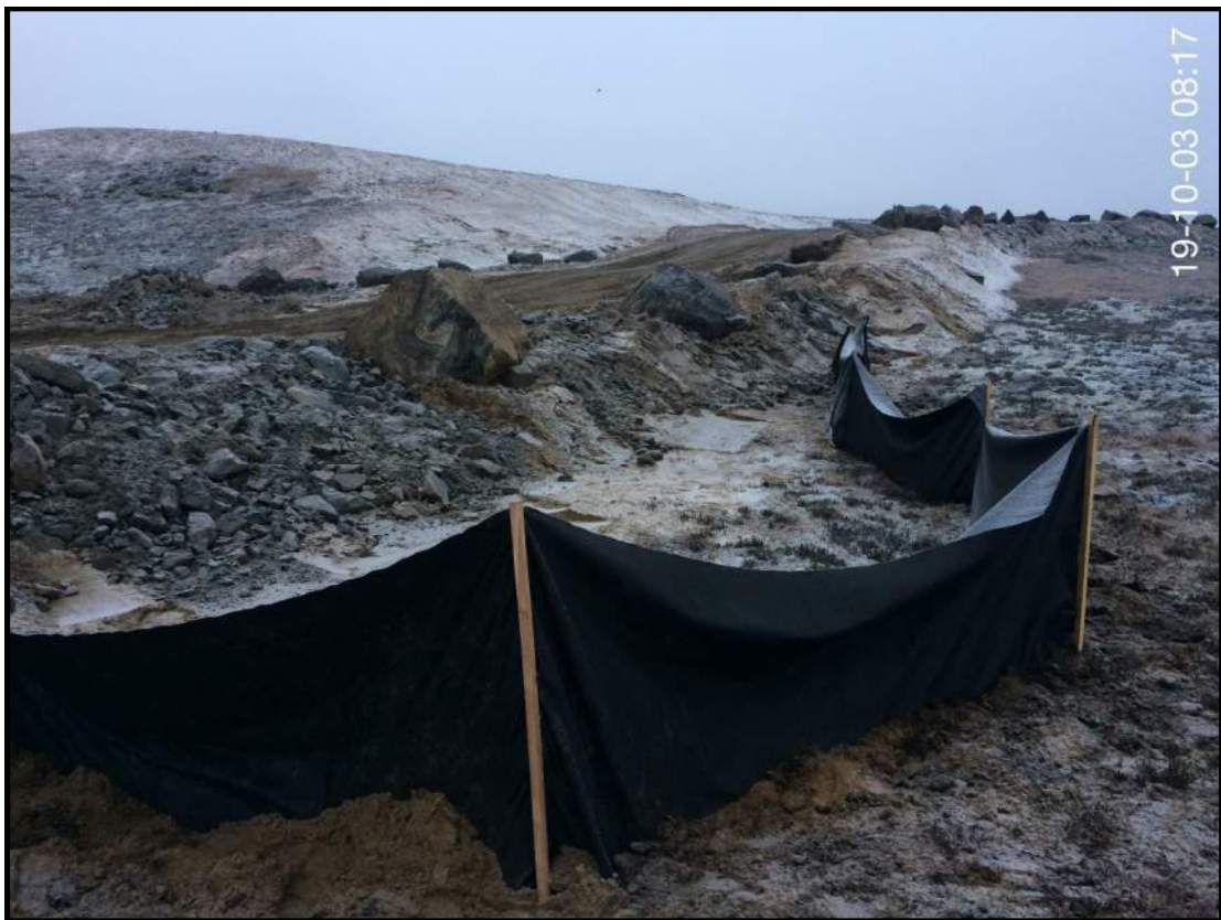
2019-10-03 CS04 DOWNSTREAM SILT FENCE
