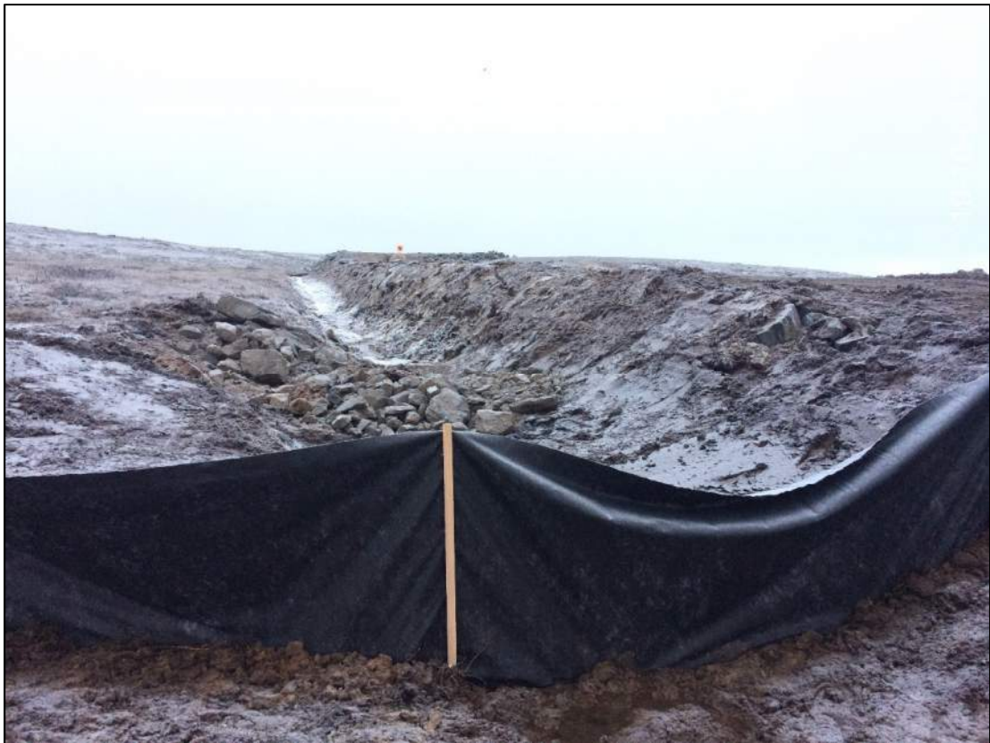
2019-10-03 CS03 UPSTREAM SILT FENCE AND SETTLING POND
