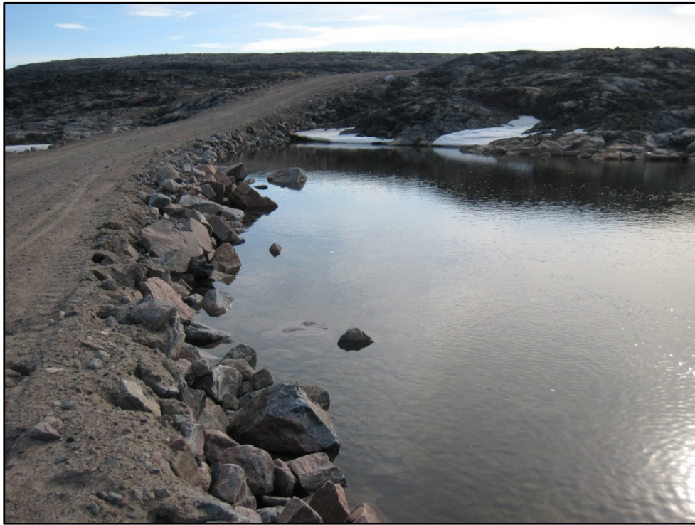
Photo 5 Substrate and large riprap of north shore of CRS-1 crossing, the freshwater lake on right side of photo; west aspect.
