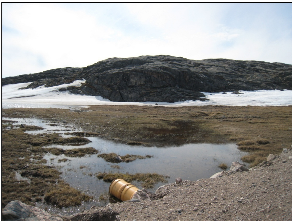
Photo 8 CRS-2 crossing west aspect with installed culvert and upstream pond flow pattern.
