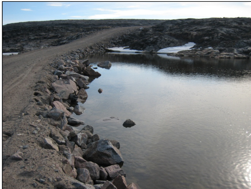
Photo 6: Tariugaq Inlet substrate and large riprap on north shore of Cross-1 in June 2008; west aspect
