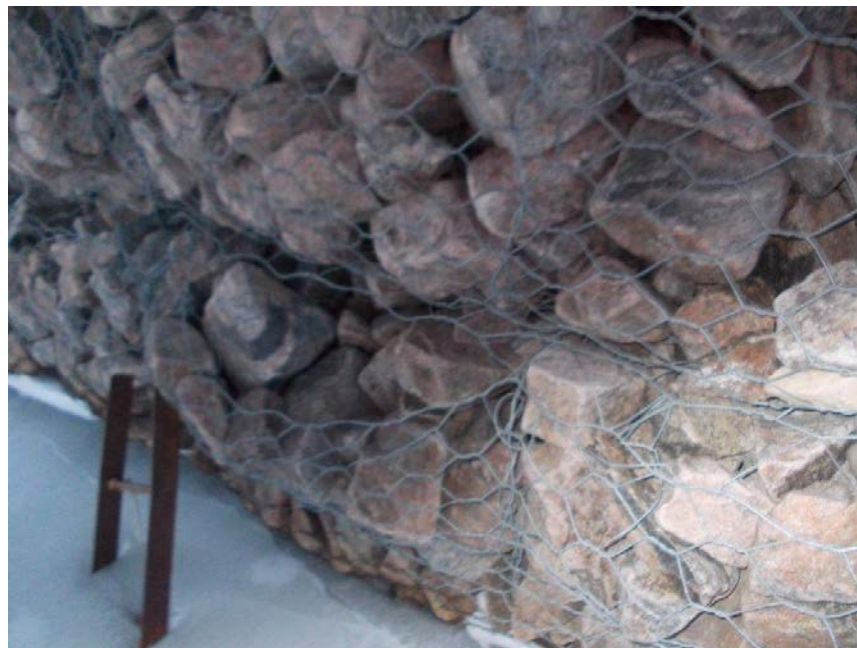
Figure 2-7: Bridge Crossing 7 – Gabions
