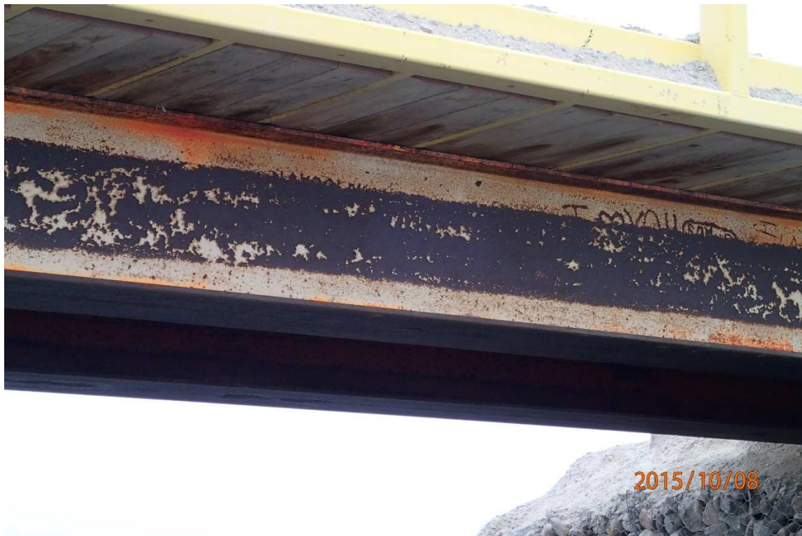
Figure 9 – Typical condition of paint coating on steel girders.
