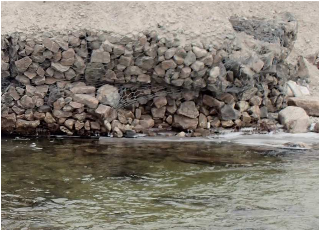
Figure 6 – Ruptured gabion basket on upstream corner of west abutment fill.
