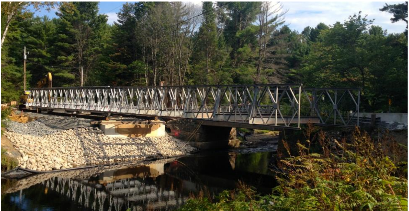
Figure 3-3: Modular Panel Bridge with Riprap Abutments
