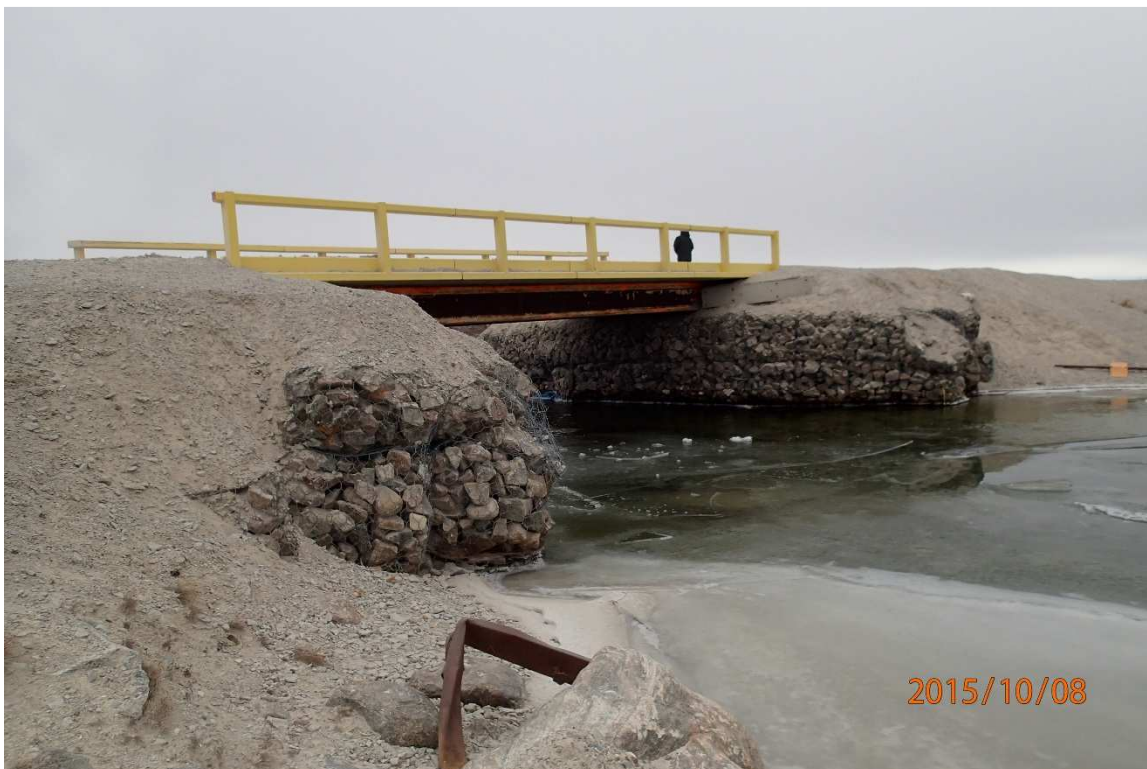
Figure 4 – East abutment gabion basket wall looking east from downstream side of bridge.
