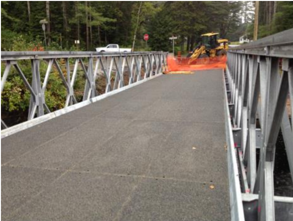
Figure 3-5: Composite Deck on Modular Panel Bridge
