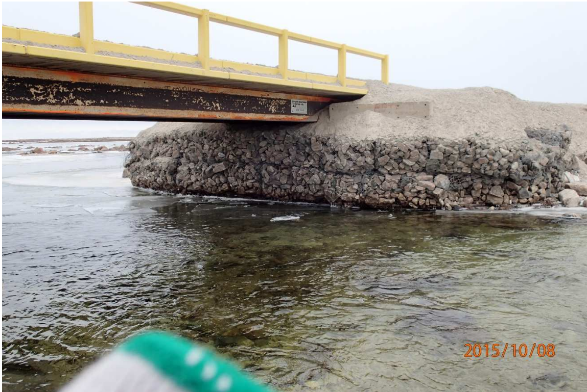
Figure 5 – West abutment gabion basket wall looking west from upstream side of bridge.
