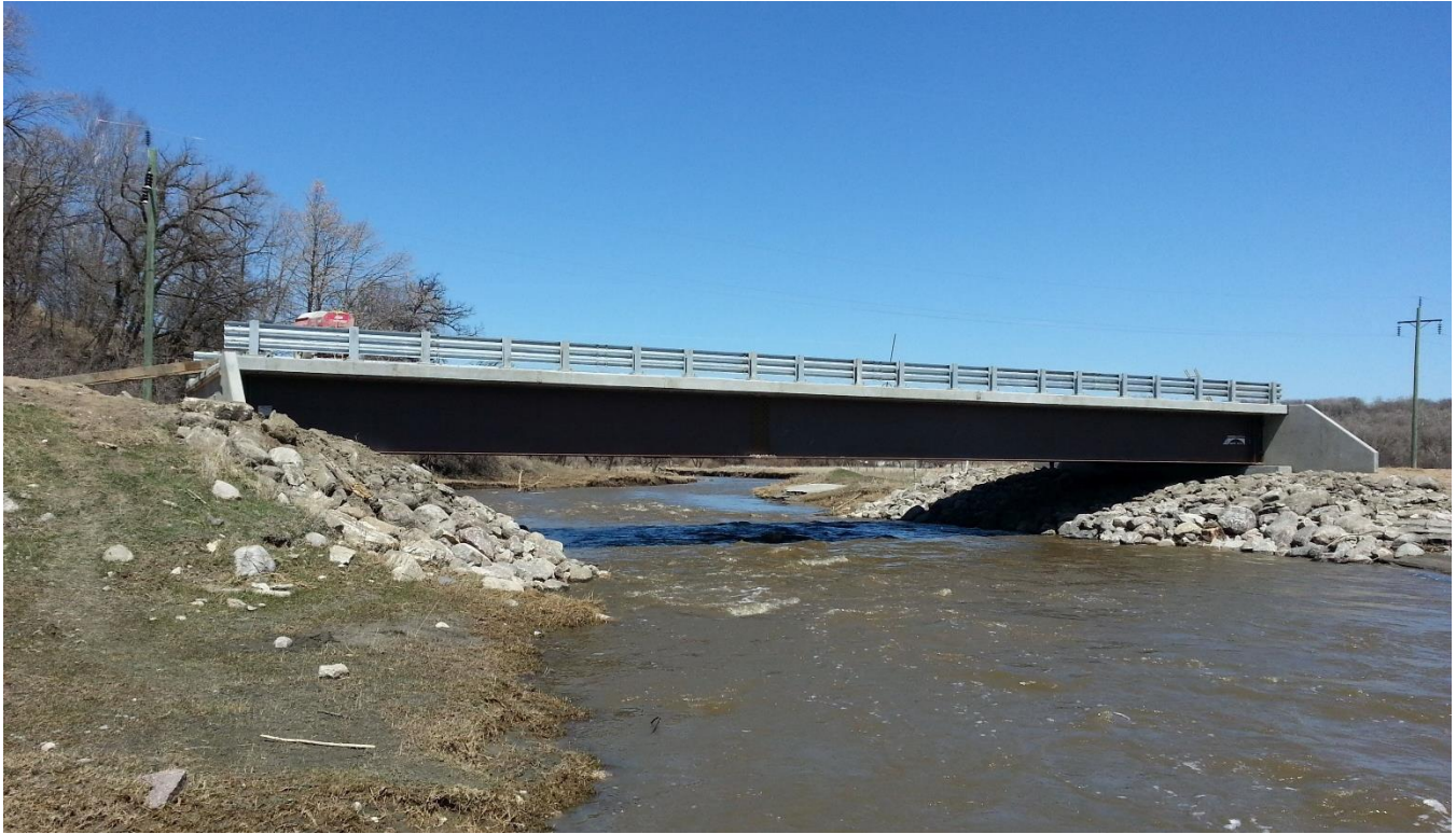
Figure 3-2: Dual Girder Bridge with Composite Deck and Sloped Riprap Abutments
