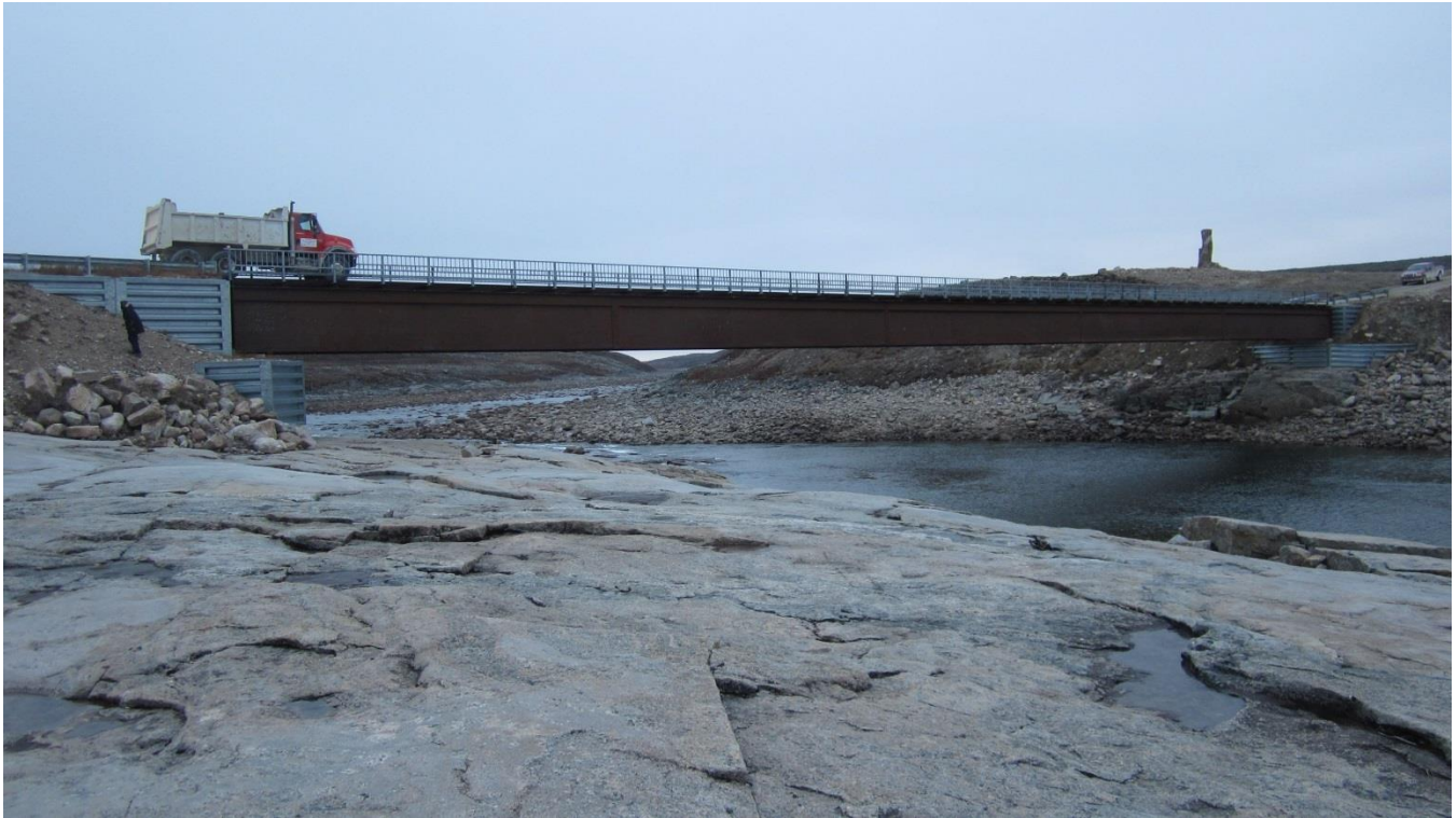
Figure 3-4: Dual Girder Bridge with Binwall Abutments (Kirchoffer River Bridge)
