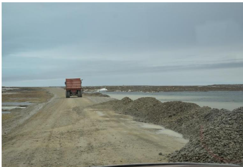
Photo 4: Fill placement along the Airport Road to help prevent it from washing out
