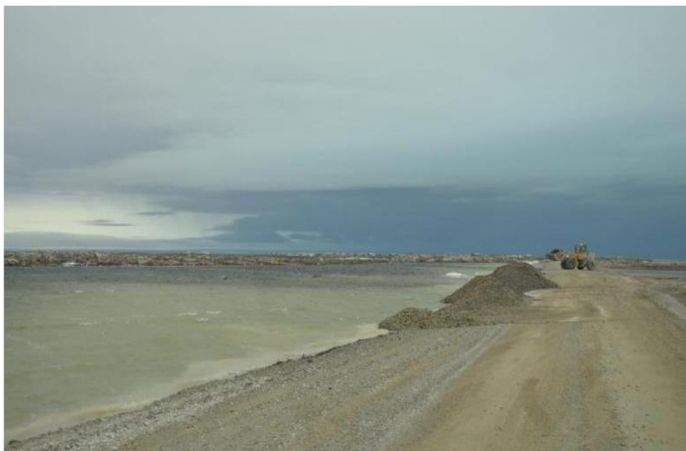
Photo 3: Fill placement along the Airport Road to help prevent it from washing out
