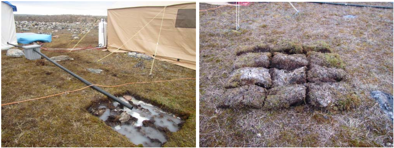
Figure 7: Draining system for greywater with grease trap (grey box) that collected all grease and debris prior to filtration through soil at location >35 m from high tide. Tundra sod (right photo) was carefully excavated, reserved, and repositioned during camp take-down in order to re-establish natural conditions at the site.
