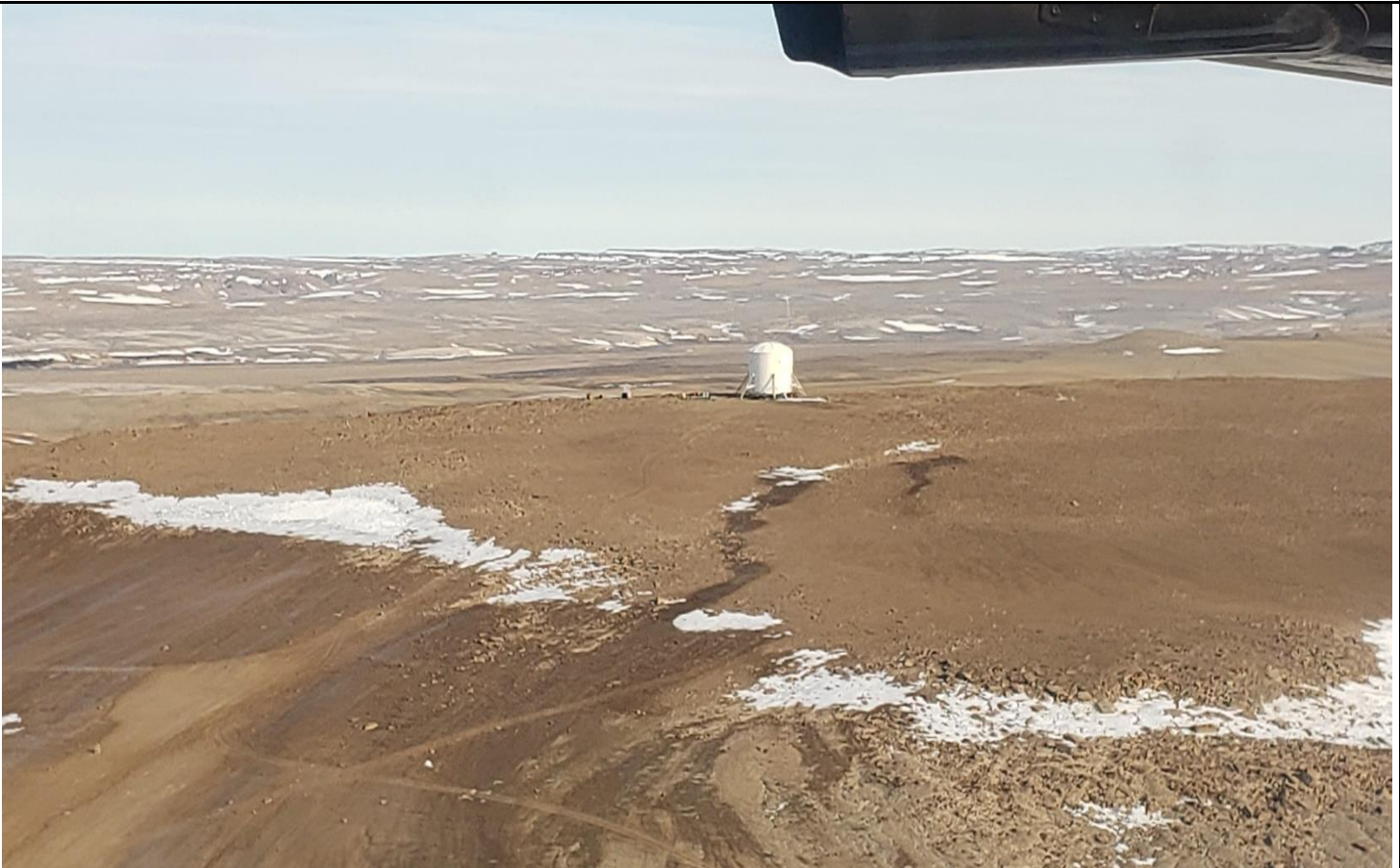
Description: Fuel cache with spill kit observed nearest to FMARS building. Yellow Spill kit with fuel cache. Waste drums on far right.
