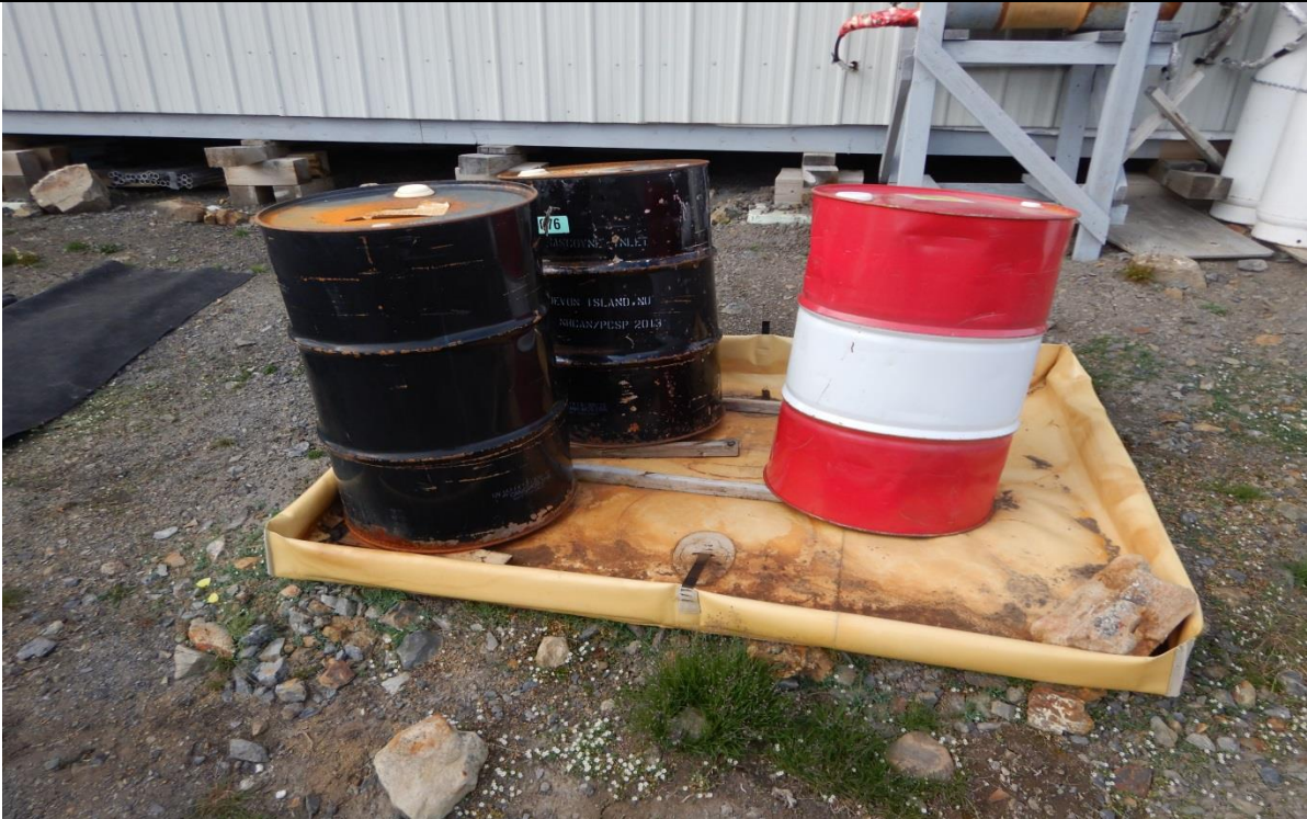
Description: 3 x drums in secondary containment.
