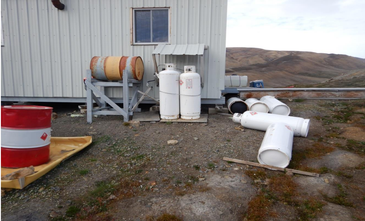
Description: building heating storage tank not in secondary containment. 7 x propane cylinders. Water storage tank next to building.
