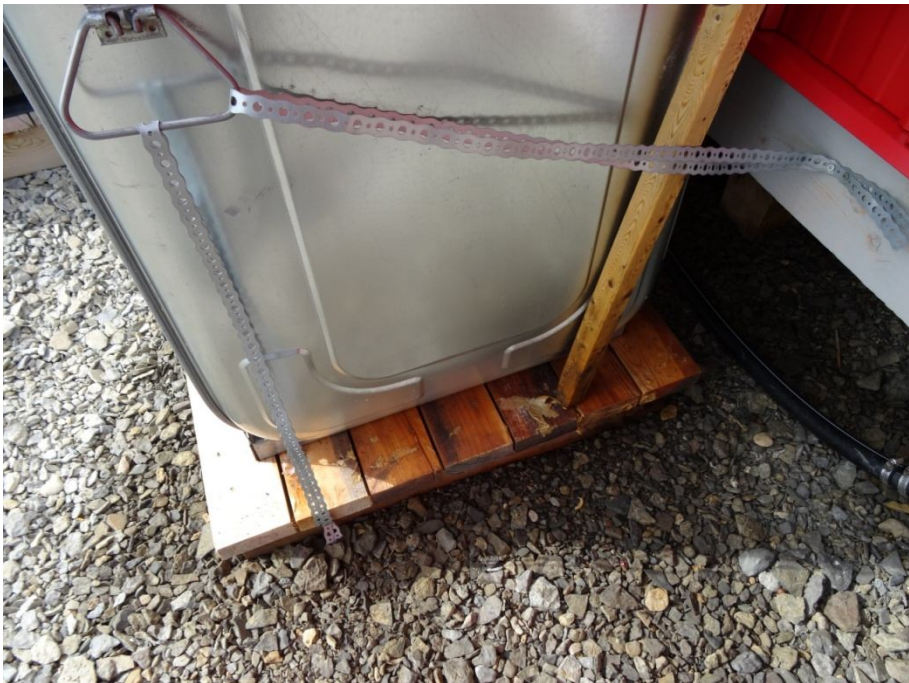
Figure 6 Tank secured to building using metal round ,, note fuel staining
