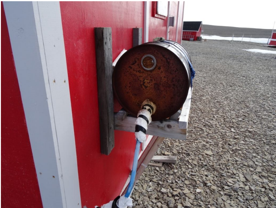
Figure 10 Fuel tank outside one of the buildings. Joints are wrapped
