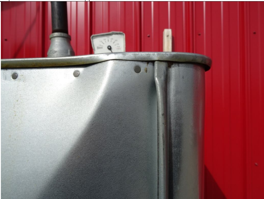
Figure 5 Fuel tank note buckled top Note rivets not welds
