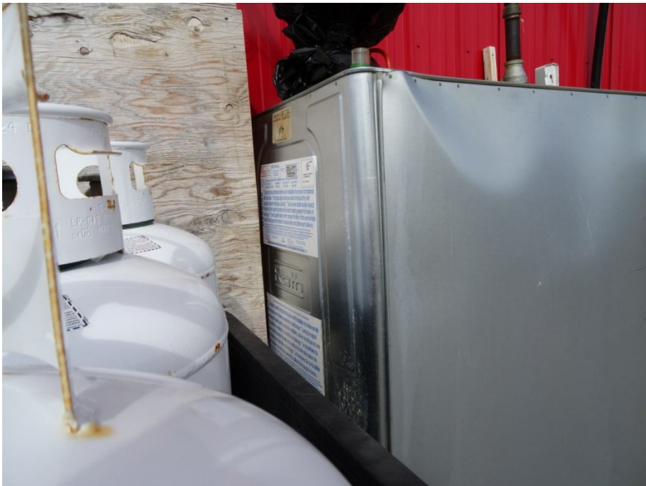
Figure 6 Tank secured to building using metal round ,, note fuel staining
