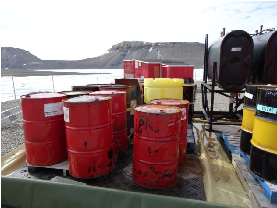
Figure 8 Fuel storage in secondary containment
