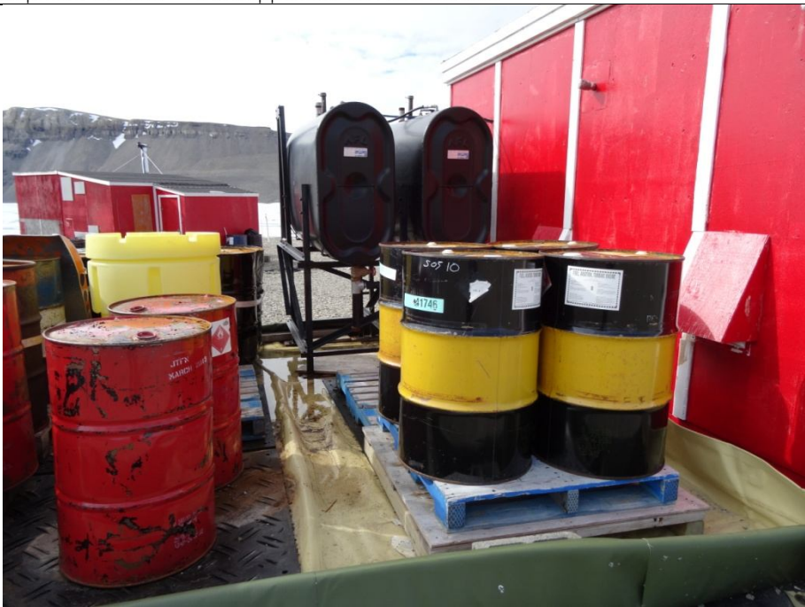
Figure 8 Fuel storage in secondary containment
