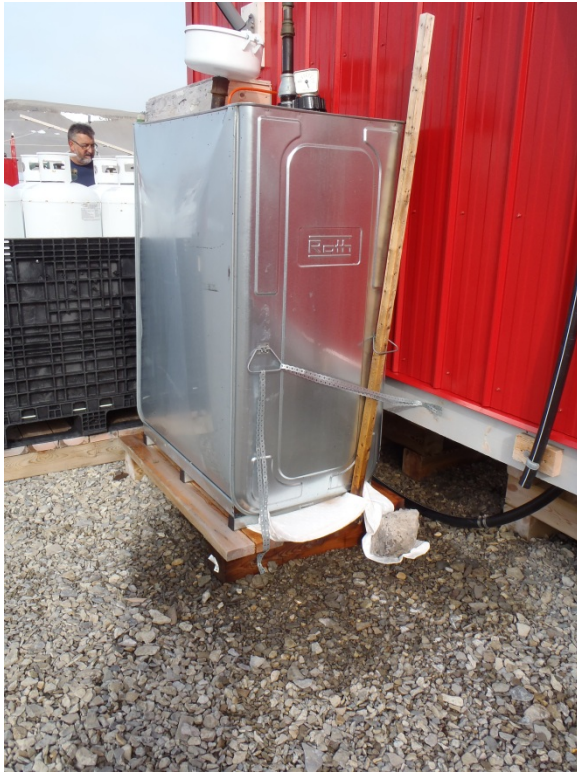
Roth tank showing bowing to outer skin
