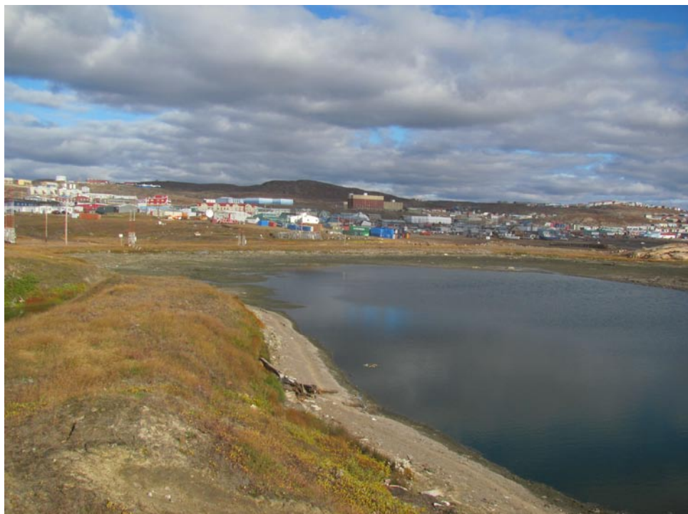
Photograph 2 Overview looking East; note lagoon level and sludge accumulation.
